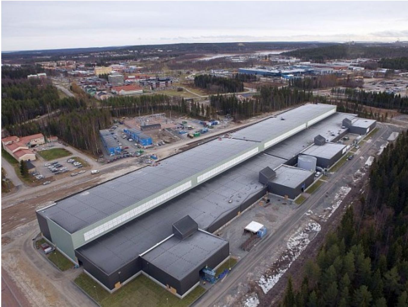
Data center, Luleå (SE), near the Arctic circle
